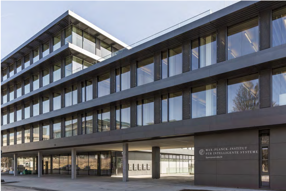
Figure 1.2: The new building of the MPI for Intelligent Systems in Tübingen.
