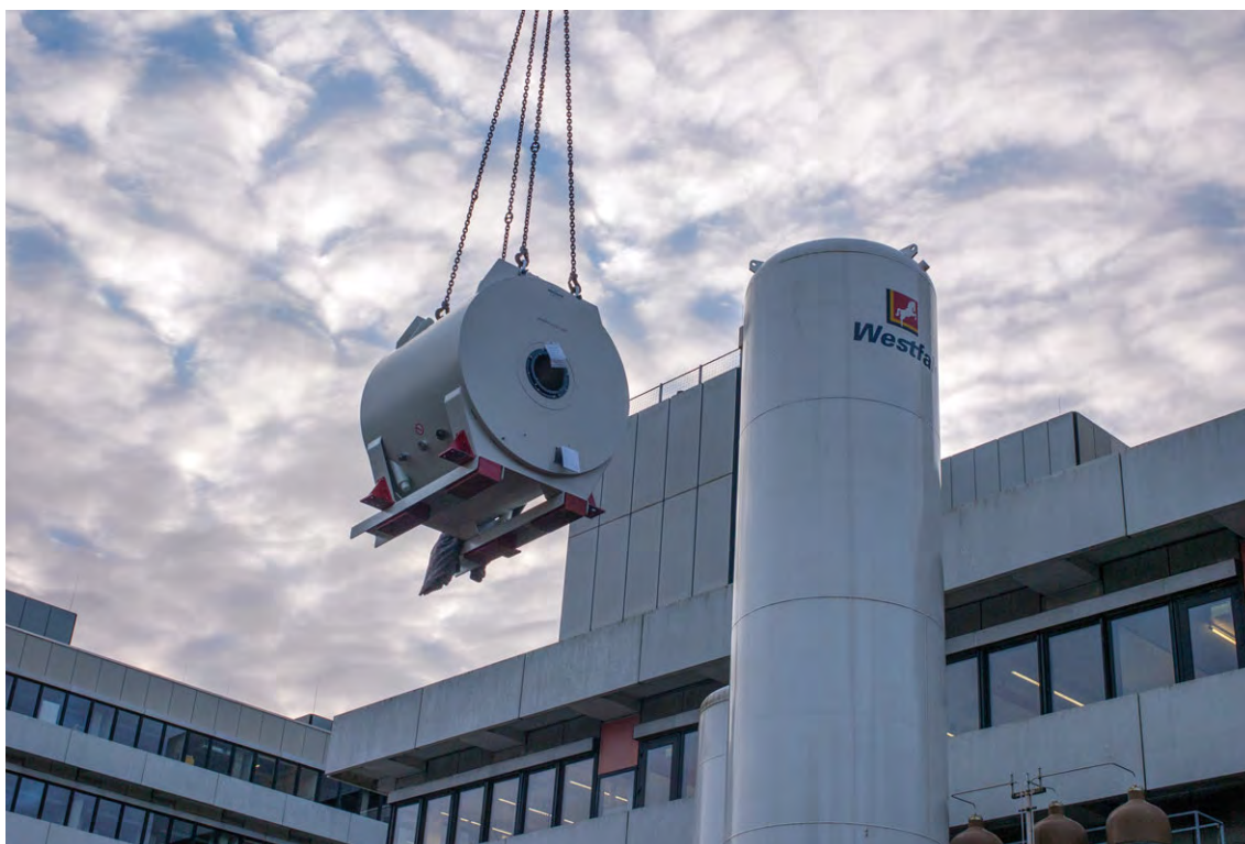
Figure 19.5: Installation of the seven Tesla preclinical magnetic resonance scanner on the MPI-IS campus in Stuttgart in January 2019.
